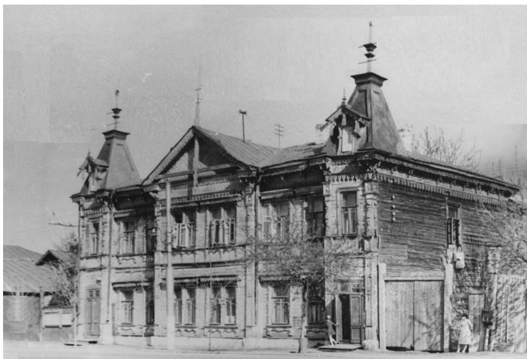
Figure 1. M.D. Mashtakov's house: street view.
