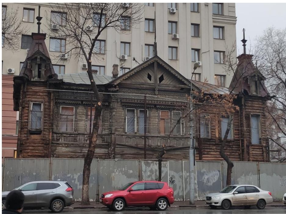
Figure 3. State of M.D. Mashtakov's house before restoration.
