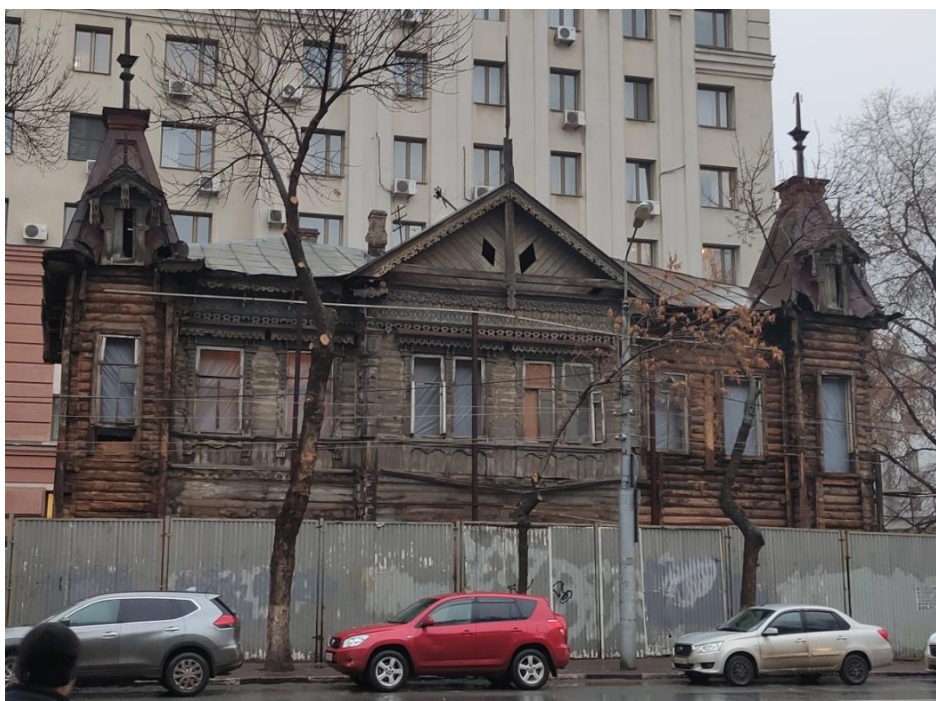
Figure 3. State of M.D. Mashtakov's house before restoration.
