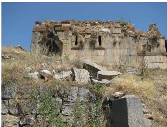
Figure 1. Neghuts monastery: view from the south.
