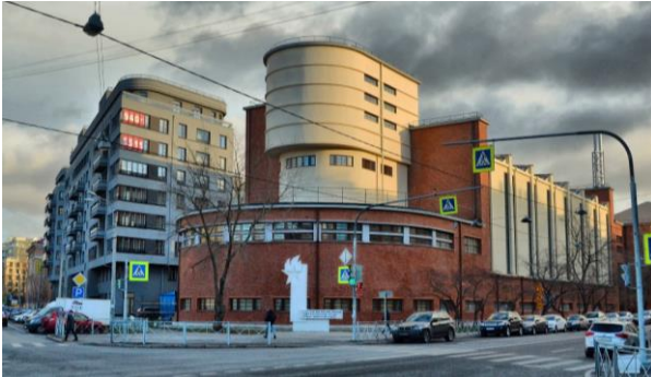
Figure 6. The Power Plant (2018 photo).
