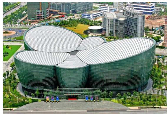
Figure 6. Center for Oriental Art in Shanghai (architect: P. Andreu).
