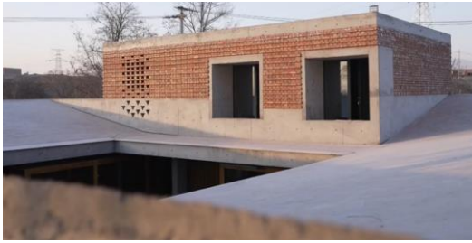
Figure 3. Roof drawing of red brick residential building in Gansu (source: Video screenshot).
