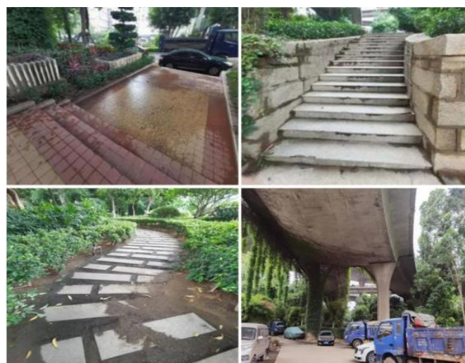
Figure 3. Current situation of the space under the Dongdu Overpass. From: author's on-site photography.
